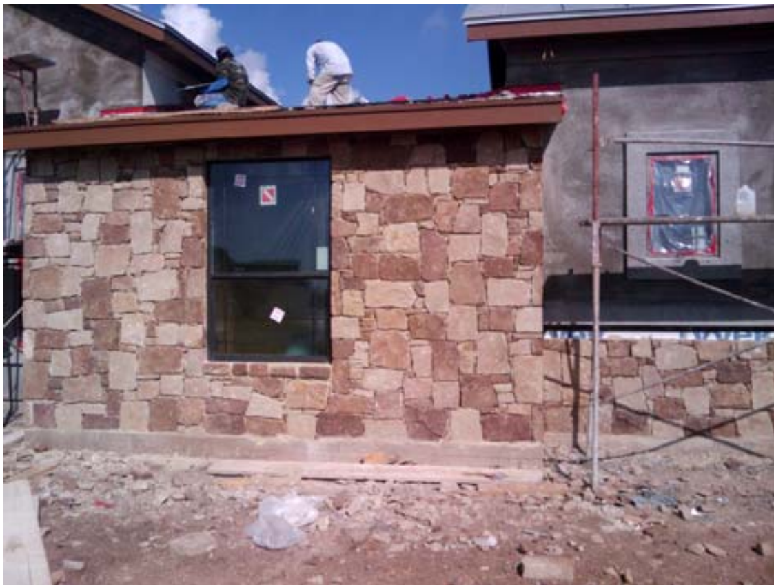
Under Construction – Nordstrom Custom Homes at 106 River Ranch Circle
