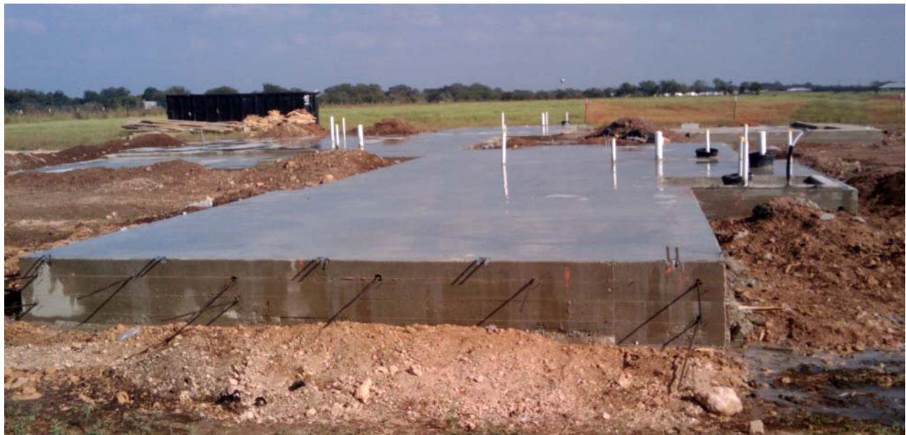
Under Construction – Nordstrom Custom Homes at 106 River Ranch Circle
